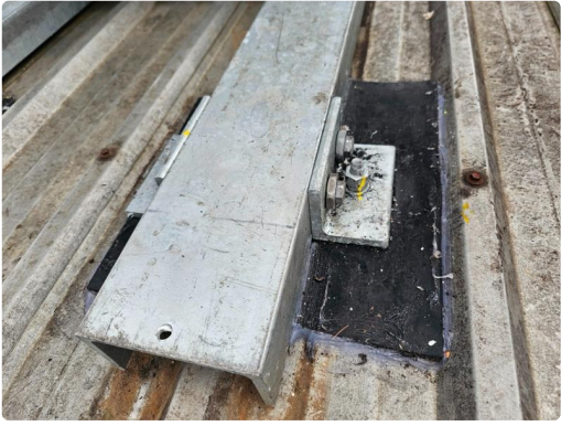
Photo 10: Site Inspection Detail (input_file_17.png)
