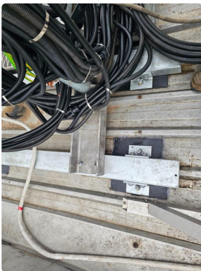
Photo 23: Site Inspection Detail (input_file_29.png)
