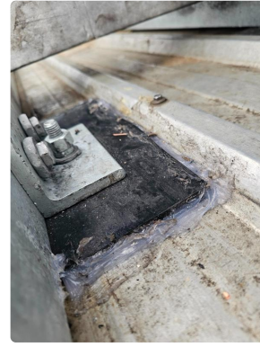
Photo 18: Site Inspection Detail (input_file_24.png)
