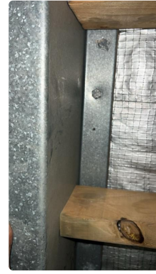
Photo 2: Site Inspection Detail (input_file_1.png)
