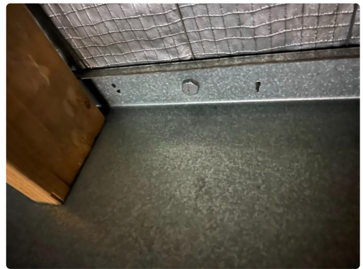
Photo 28: Site Inspection Detail (input_file_7.png)
