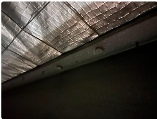
Photo 27: Site Inspection Detail (input_file_6.png)
