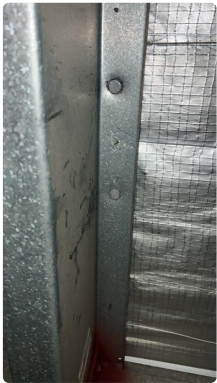
Photo 13: Site Inspection Detail (input_file_2.png)
