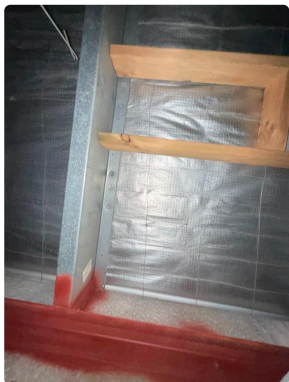
Photo 5: Site Inspection Detail (input_file_12.png)
