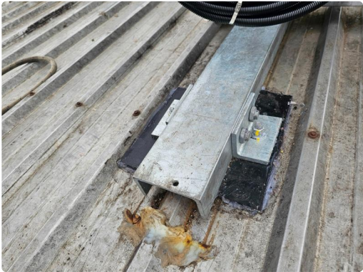
Photo 15: Site Inspection Detail (input_file_21.png)
