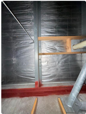
Photo 3: Site Inspection Detail (input_file_10.png)
