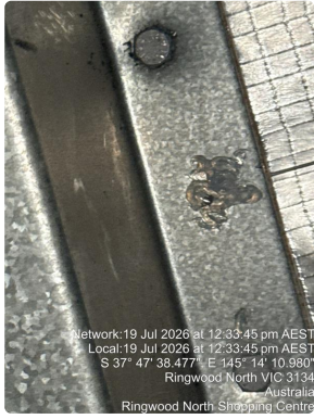
Photo 1: Site Inspection Detail (input_file_0.png)
