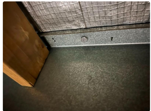
Photo 24: Site Inspection Detail (input_file_3.png)
