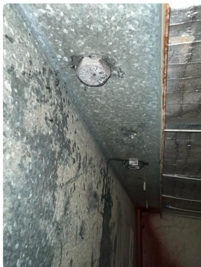
Photo 29: Site Inspection Detail (input_file_8.png)
