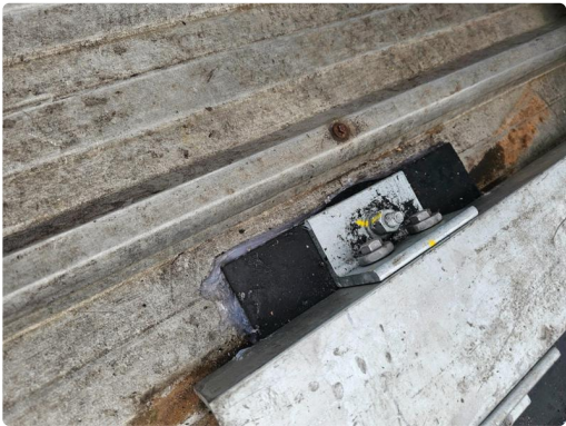
Photo 11: Site Inspection Detail (input_file_18.png)
