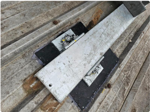
Photo 12: Site Inspection Detail (input_file_19.png)
