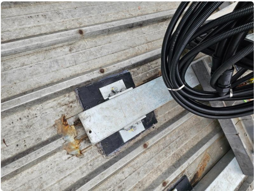
Photo 14: Site Inspection Detail (input_file_20.png)
