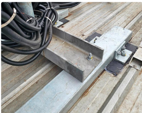
Photo 7: Site Inspection Detail (input_file_14.png)
