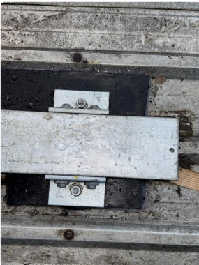
Photo 21: Site Inspection Detail (input_file_27.png)
