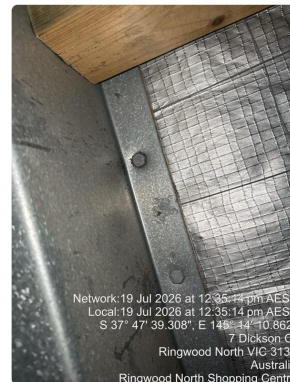
Photo 6: Site Inspection Detail (input_file_13.png)
