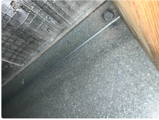
Photo 25: Site Inspection Detail (input_file_4.png)
