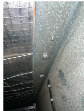
Photo 30: Site Inspection Detail (input_file_9.png)
