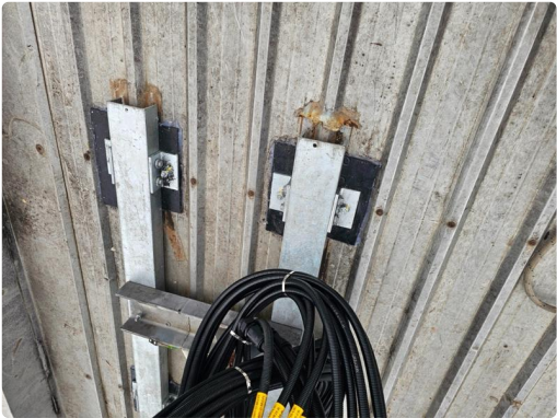
Photo 16: Site Inspection Detail (input_file_22.png)
