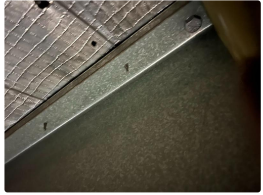
Photo 26: Site Inspection Detail (input_file_5.png)
