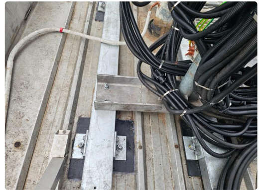
Photo 20: Site Inspection Detail (input_file_26.png)
