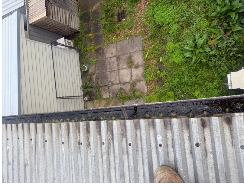
Photo: Gutter line and roof edge condition from above (inspection media folder 2).
