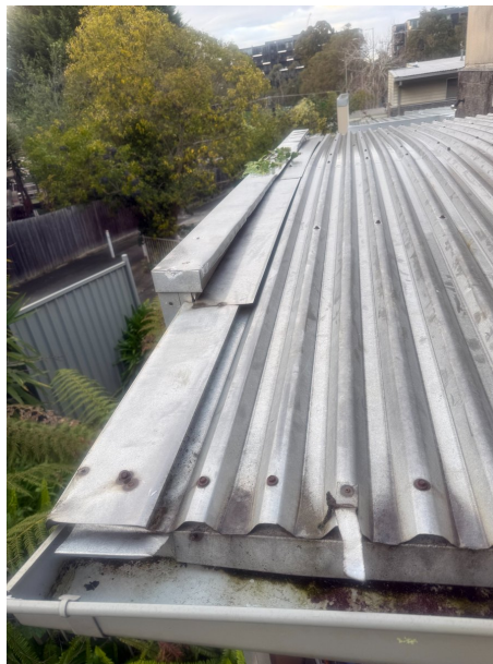
Photo: Edge detail, barge and gutter junction (inspection media folder 5).
