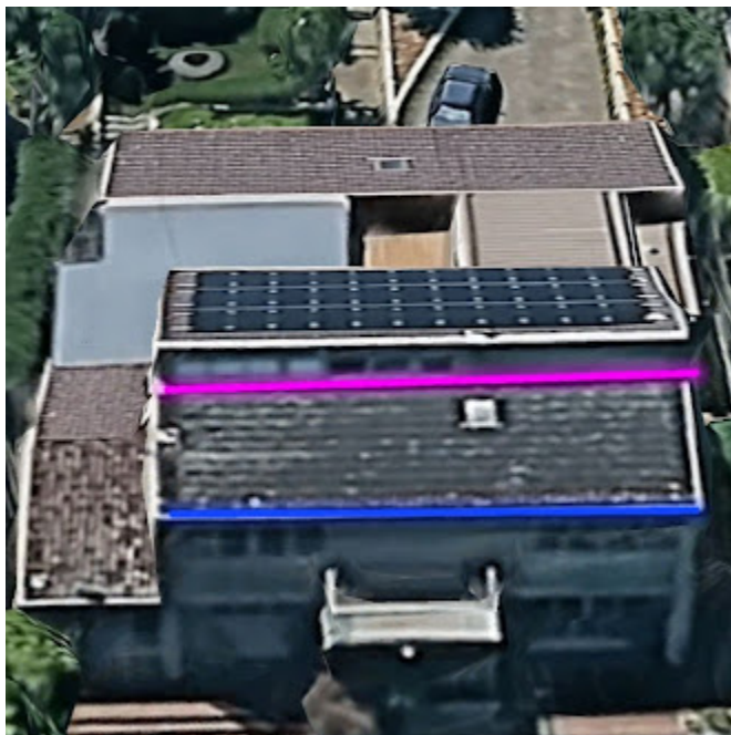
Close-up Highlighting Blue (Box Gutters 25 m Total) Areas Here]
