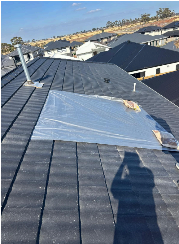
Completed make safe. Heavy-duty tarp secured with sandbags to prevent further water ingress
