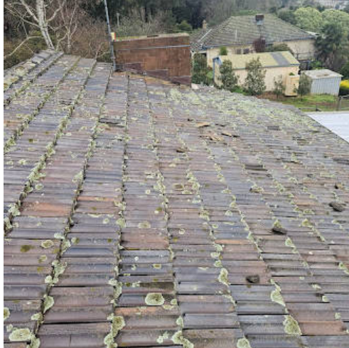
Picture 2: Indicates dirty roof and moss on roof that will require to be hi pressure cleaned rubbish removed and broken tiles changed.
