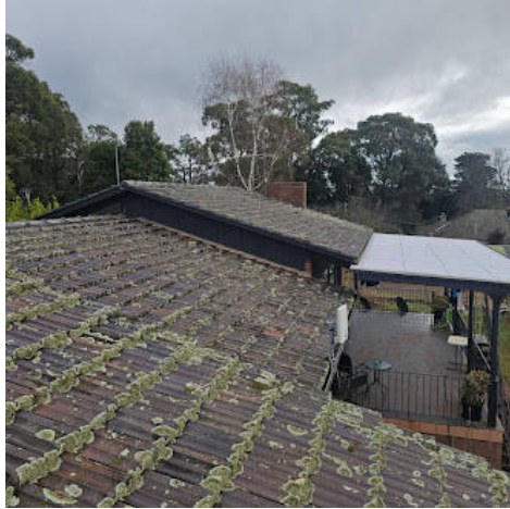
Picture 6: Different angle of roof that shows how dirty the roof is with moss growing on it that will require high pressure cleaning.
