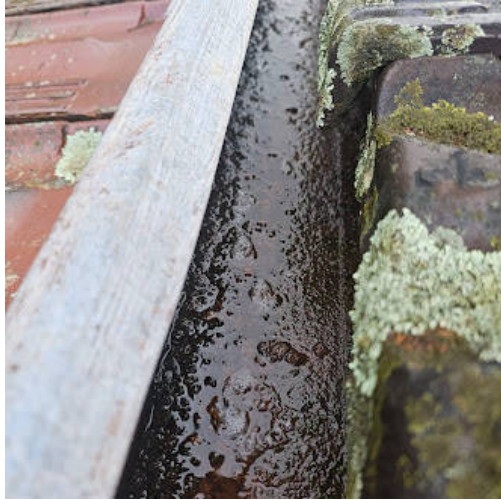
Picture 8: Showing gutters and flashings in poor condition that will require to be changed due to rust and water leaks.
