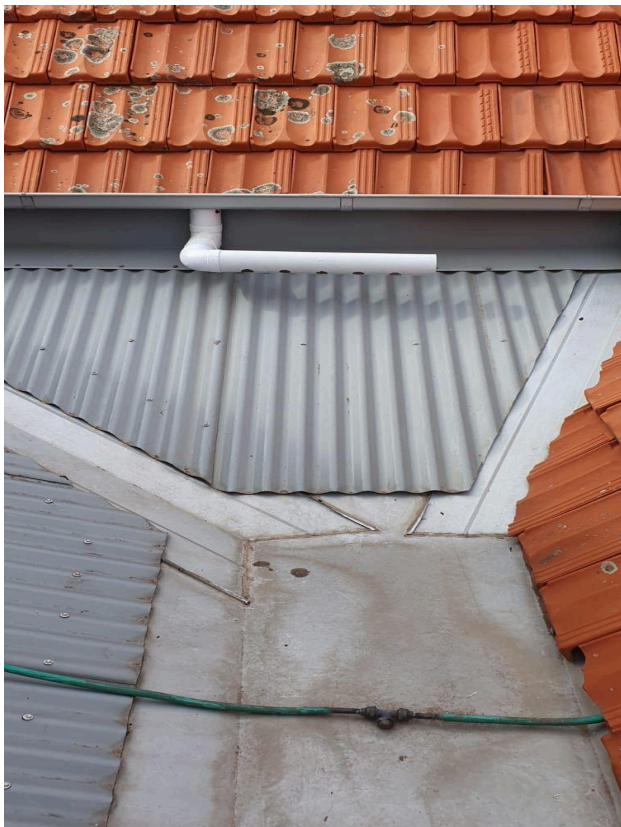
New Photo Attached: Spreader Installed
